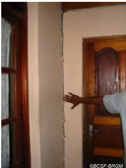
Fig. IV-73. Bouillante - quartier Courbaril - large fissuration.
