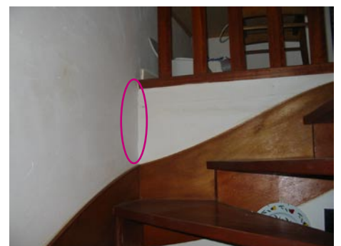
Fig.21 - fissure intérieure (Kerhen-Liven, Languidic).
